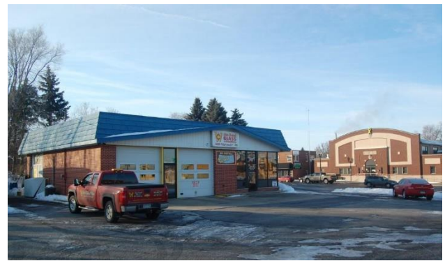
Current business on the southwest corner of Broadway Street and 3 rd Avenue (will become part of the Site).
